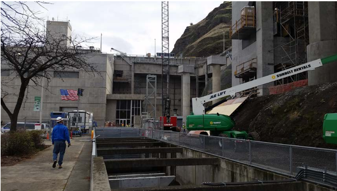
Photo 1. Installation of the above ground temporary potable water line and connection to the existing water line will occur on the north side of the ladder.
